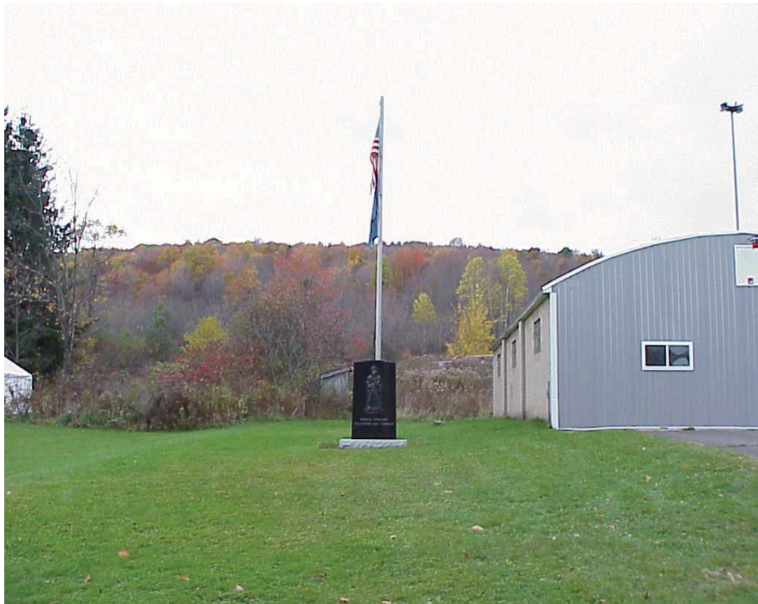
View of Warren Township Volunteer Fire Department.
